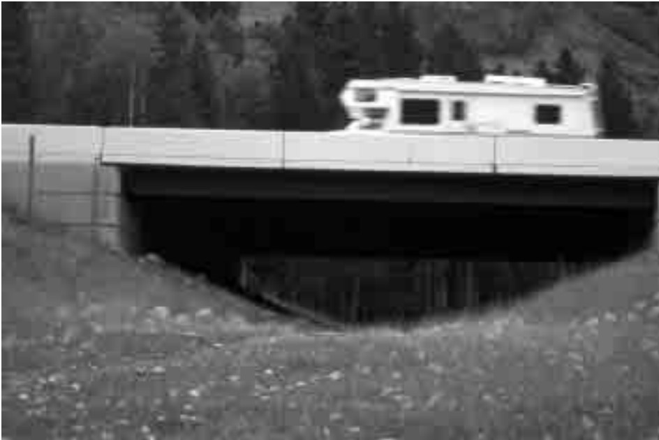
Fig. 5-2 (a) Highway underpasses combined with roadside fencing have greatly reduced the number of Elk killed on the trans-Canada highway in Banff National Park, Canada. (Photo: A. Bennett).
