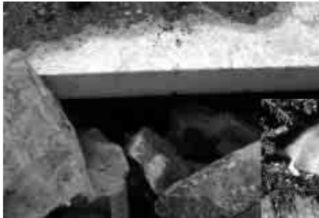
Rock-scrree corridor and tunnel for the Mountain Pygmy-possum in Australia
